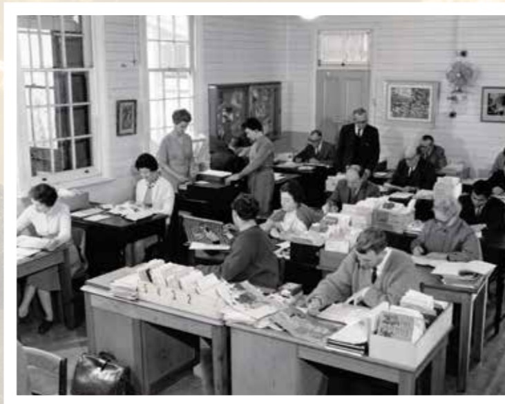
Art Department in the "portable" building at Blackfriars
